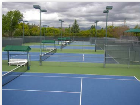
New Courts! Court renovation almost complete.
